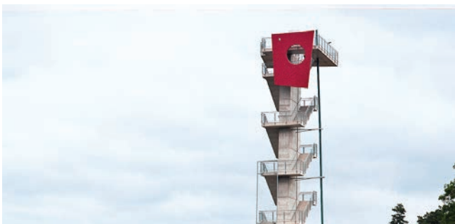
coal mining viewing tower
