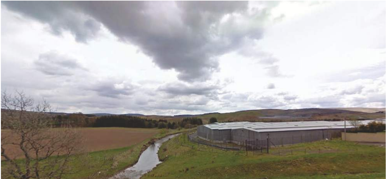
the former Ramage's premises at Glespin
